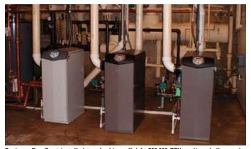
Designer Don Smet installed two Lochinvar Knight 500,000 BTU mod/con boilers and a Lochinvar Armor mod/con water heater with 399,000 BTU together in the main building. Photo courtesy of Lochinvar.
